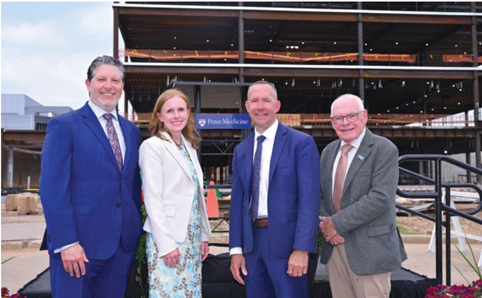
Penn Medicine Princeton Health celebrated a major construction milestone this summer: topping out its $401 million Penn Medicine Princeton Cancer Center project. Located on the Princeton Medical Center campus in Plainsboro, the cancer center includes a six-story parking garage that opened in July 2025. It is the largest expansion of Princeton Health since the hospital relocated from Princeton in 2012. Once completed in May 2028, the facility will house more than 40 exam rooms, 30 infusion chairs and two linear accelerators; as well as a breast imaging center and advanced diagnostic technologies including CT, MRI, and SPECT/CT. Princeton Cancer Center will target LEED Gold certification. It will incorporate green roofs across all canopies to minimize the heat island effect, and rain gardens will capture excess water run-off.
