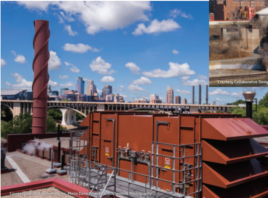
Courtesy Jacobs Engineering Inc. Photo Dana Wheelock, ©Wheelock Photography.
