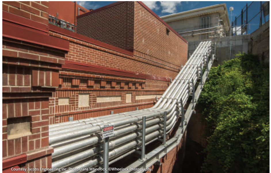
Courtesy Jacobs Engineering Inc. Photo Dana Wheelock, ©Wheelock Photography.
